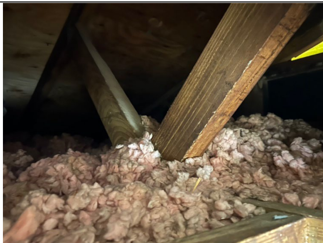
FIBERGLASS ATTIC INSULATION
