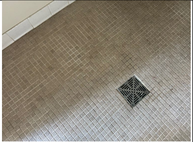
GROUT/MORTAR 1"X1" CERAMIC FLOOR TILE - OFFICE BATHROOMS
